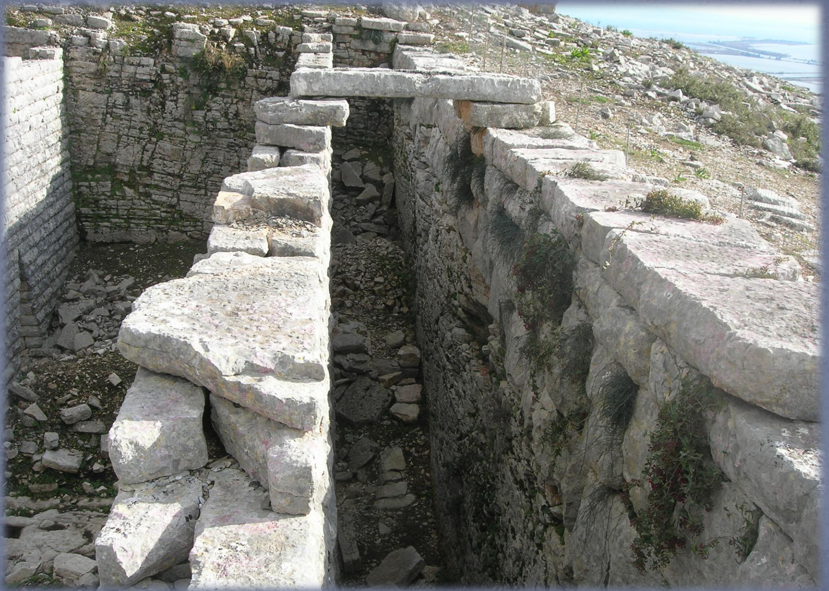
The south compartment with the original roofing
